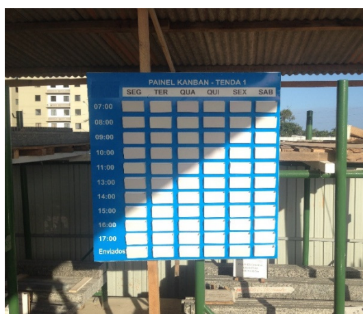
Figura 3 – Painel kanban na central de kits
