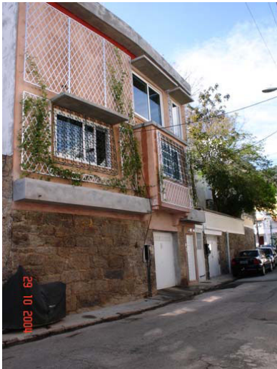
Fig. 14 – Fachada NO com as trepadeiras
