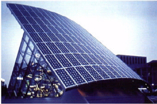
Figura 2: The Solar Showcase. Port Talbot, UK. 15 kWp instalado.
