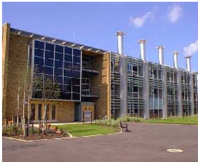
Figure 11: The BRE headquarter
