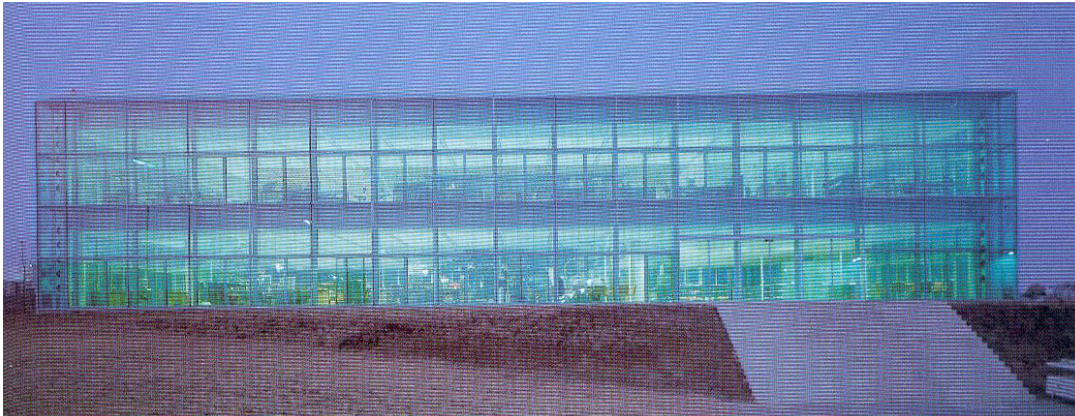
Figure 8: Administrative building in Würzburg
