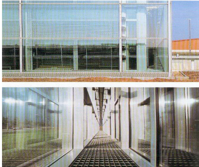
Figure 10: Double façade design
